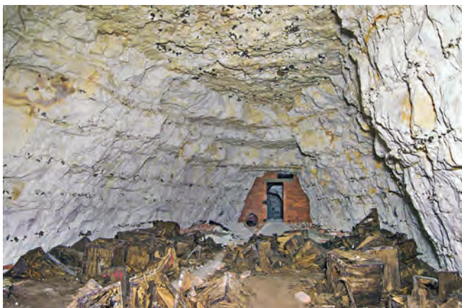
Looking from the main repository chamber towards its entrance brick screen. The peculiar large diameter pipe passing through the wall resembles the large sewer pipes used in Stockport's Chestergate shelter, but the function here is likely to have been for ventilation
